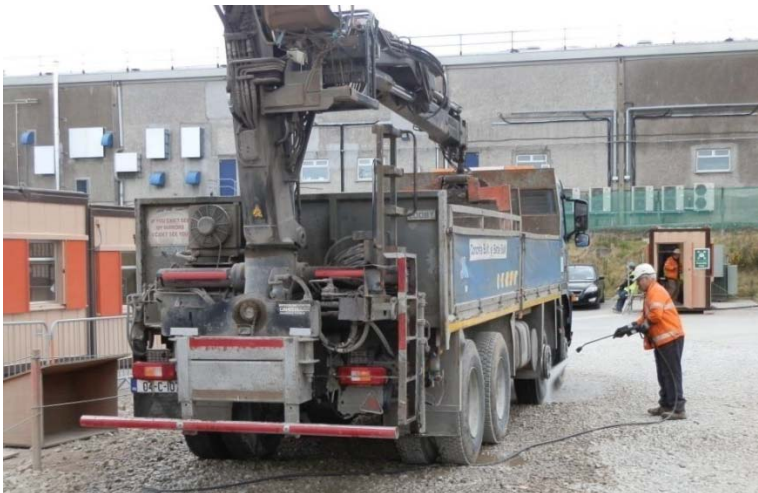
Figure 6.3 – Example of wheel washing of truck as it leaves site
